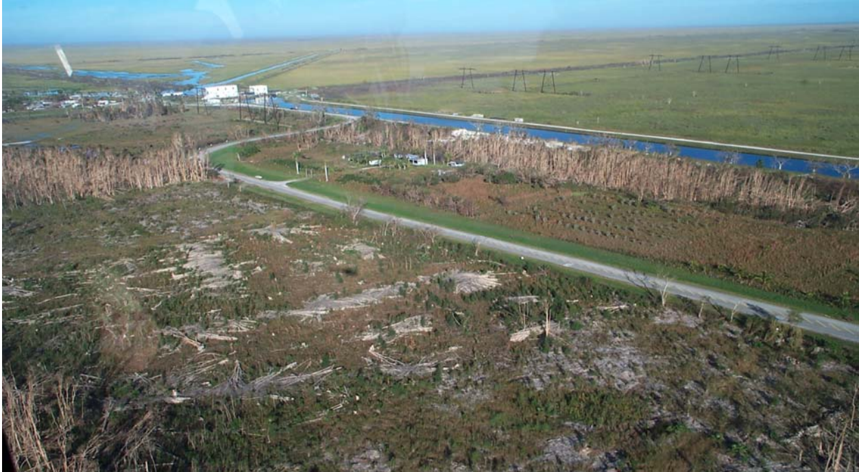
Figure 1: Looking North along the C-11 Canal towards Water Conservation Area 3A and pump station S-9.
