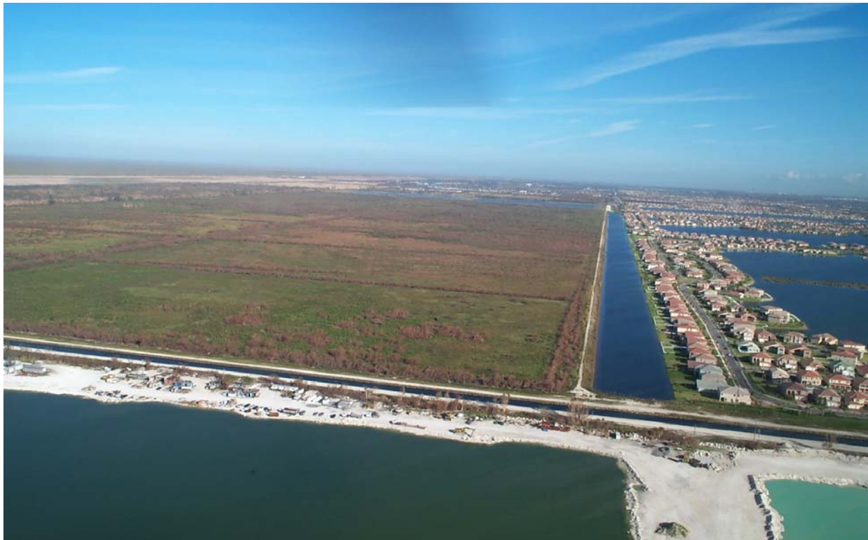
Figure 2: Looking North across Broward County WPA project across C-9 canal and the future location of the C-9 Impoundment.
