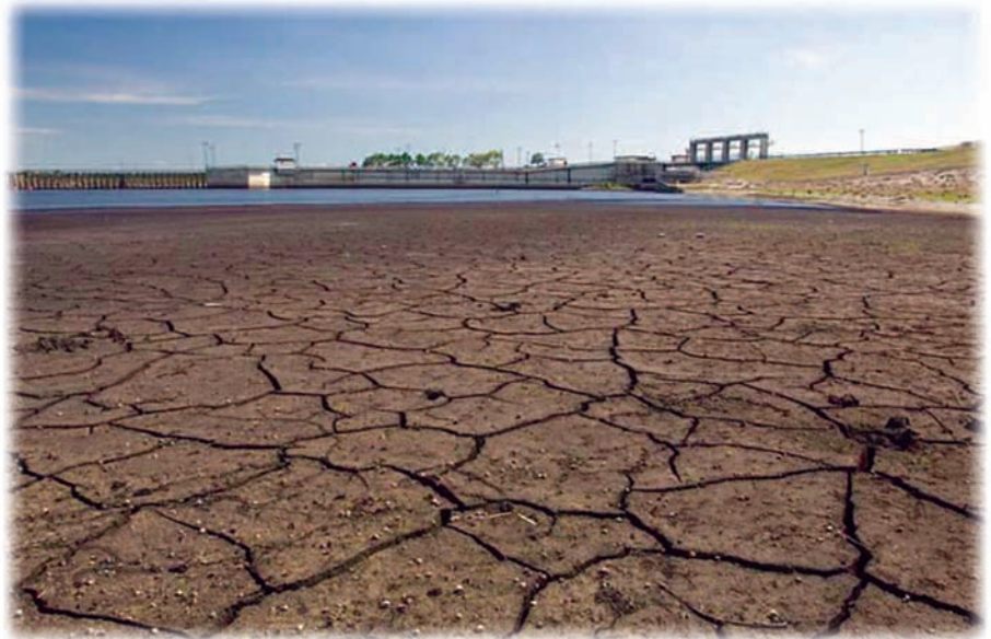
Many miles of dry lakebed was exposed in the spring of 2007. This photo was taken on the east side of Lake Okeechobee, near the S-306 structure in Port Mayaca.
